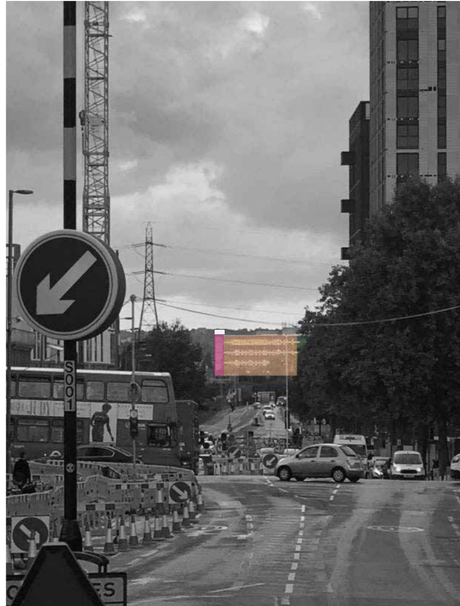
view from Blackhorse Road
